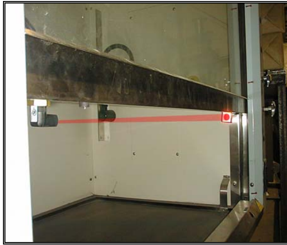
Figure 9 - The Photoelectric Sensor Emits a Point Source of Light that is Bounced Back by the Reflector on the Opposite Side of the Sash. The Beam is not Visible and Has Been Added to this Picture.
