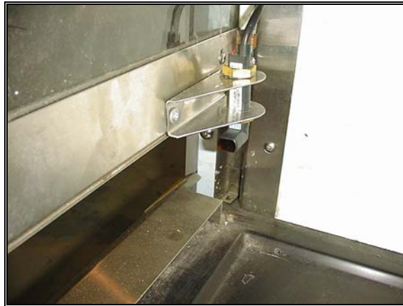
Figure 6 - Photoelectric Sensor Attached to the Bottom of the Sash
